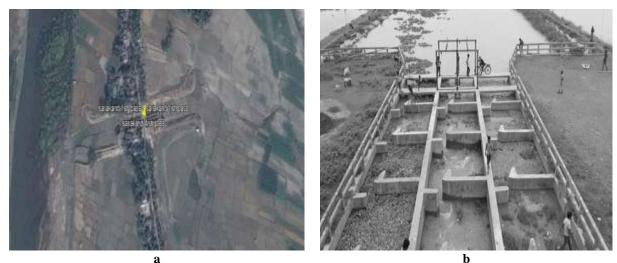
Fig. 2. View of the study site: a. Aerial view; b. Vertical slot type fish pass.
