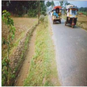
Fig. 13. Public roadsides being damaged by irrigation canal. RAMPT models may be followed to save the roadsides
