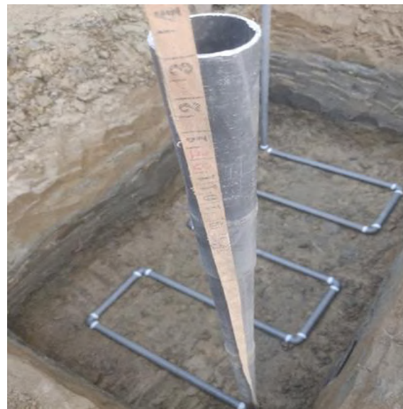
Figure 3: Pipe loop installation for EWPHE system
