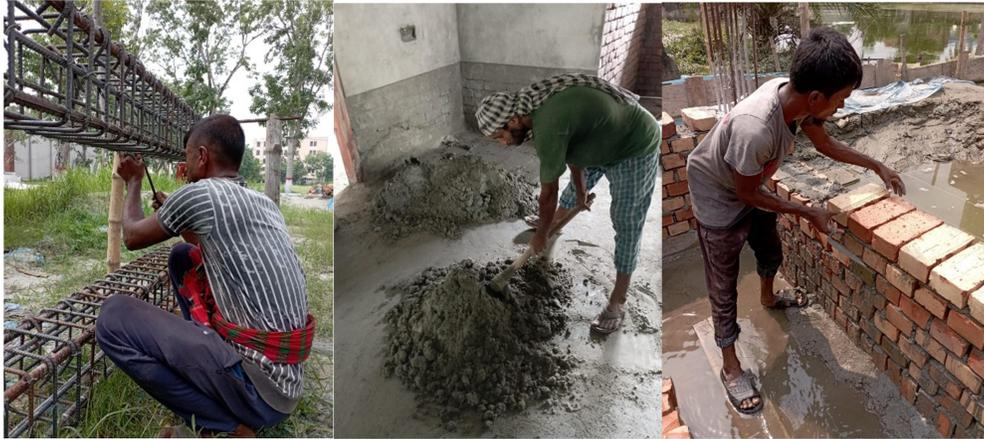
**Figure 1:** Workers doing Beam and column casting (Left side), Sand and cement mixing (Middle) and Masonry (Right side) work in awkward posture.
