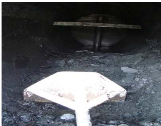
Fig. 9. Reboiler inside condition
