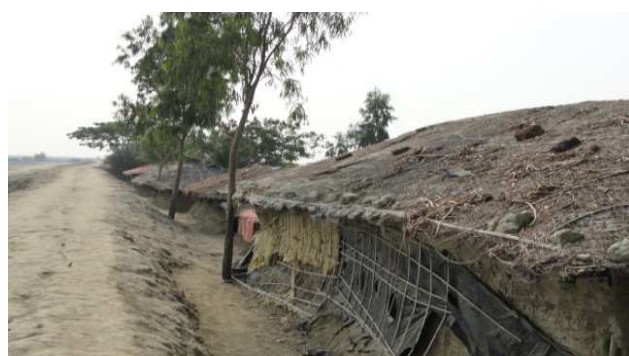
Fig. 2. Location of House by Side of Embankment, Kutubdia, 2010
