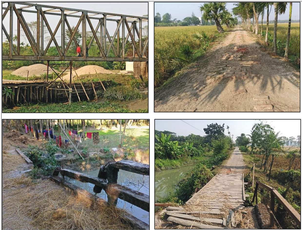
Figure 6: Unimproved and Deteriorated Roads in the Study Area (Upper Left: Flimsy Bridge at Arpangashia, Upper Right: Dilapidated Brick Paved Road in Naltona, Lower Left: Broken Guard Rail on a Buckling Bridge at Char Kalmi, Lower Right: Makeshift Bridge at Naltona Near Bishkhali River)
