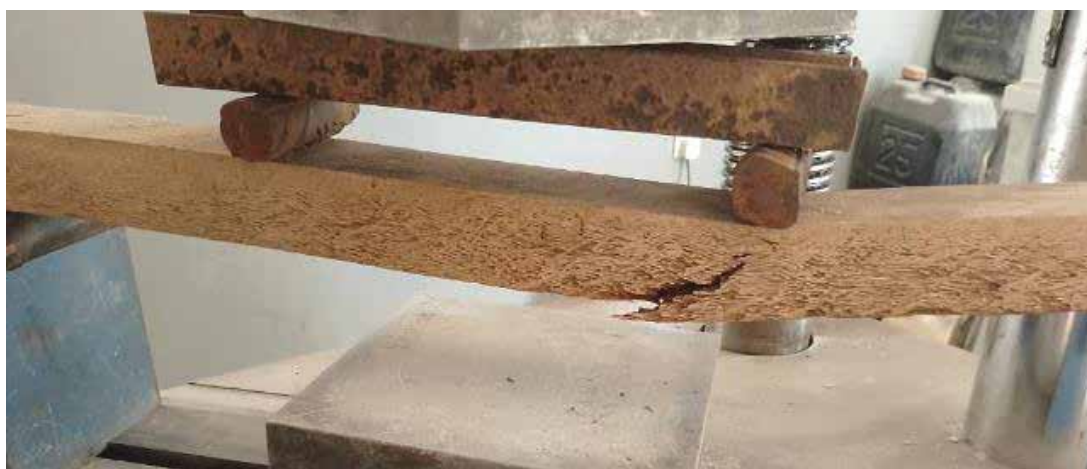
(a) Solid coconut beam failure
