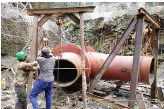
Fig. 22. Bifurcation during installation
