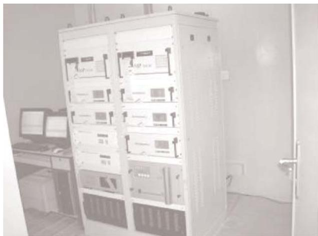
**Fig. 1: Multiple Gas analyzers inside of CAMS**
